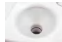
Sewage Drain Outlet
